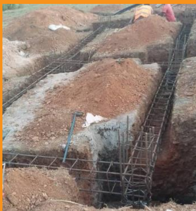
Construction of 30 cubic water tank
